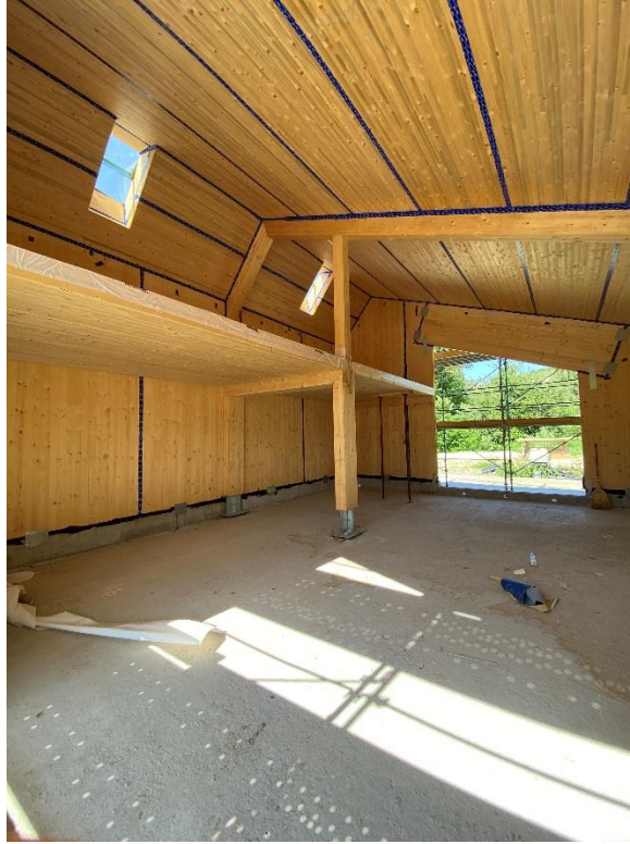
Figure 23 Internal view of one of the buildings
