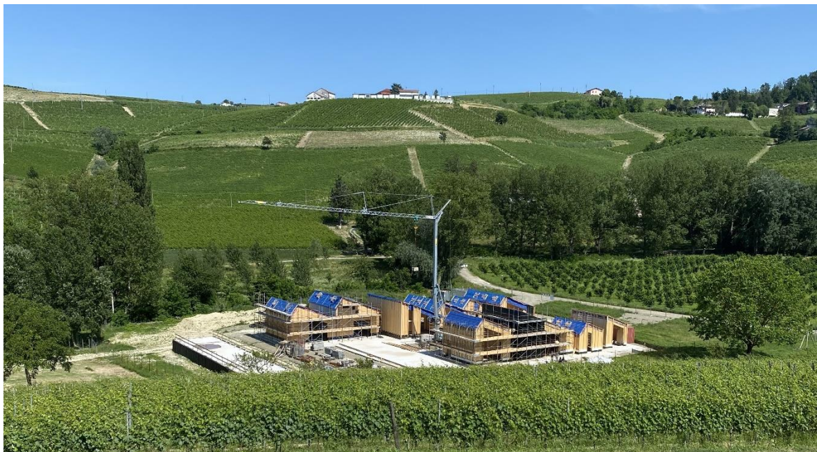
Figure 12 Buildings under construction
